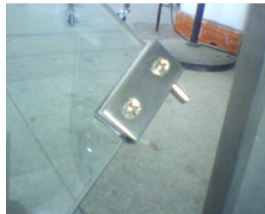
1. Lower left side door hinge assembly with two gaskets as above. Install the door hinge to the lower left side of the glass door, paying particular attention to the white colored gasket. The gasket must be placed on the screw side of the door hinge between the glass and the door hinge itself. The other gasket is to be placed on the outside of the door hinge in between (in the same manner). Please note do not over tighten the screws as this can lead to damaging the glass door.
